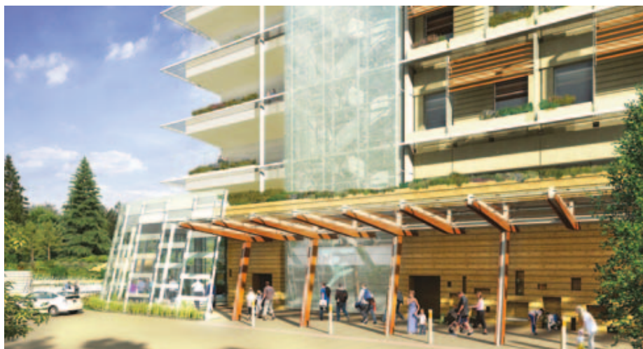
Lucile Packard Children's Hospital in Palo Alto, California, is collecting, storing, and using rainwater for irrigation onsite. Rendering courtesy of HGA Architect and Engineers
